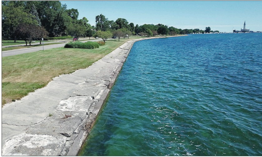
DRONE PHOTO COURTESY OF SKY TECH
